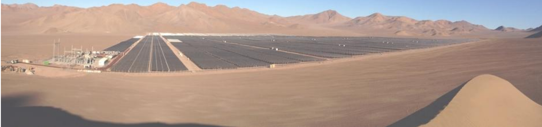
General view of the “Amanecer Solar CAP” Plant site, as of March 2014
